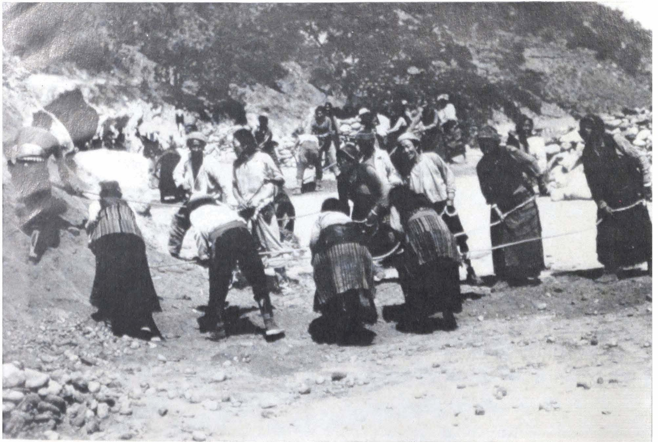
Road-workers' camp, Kulu Tibetan road workers moving rocks by hand
